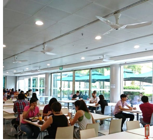
Bosch Singapore cafeteria, 2017. Photo: Bosch Fans cool first, then run together with air conditioning above 79°F (26 °C).
