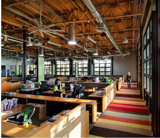
DPR Construction, Phoenix AZ, 2011. Photo: DPR Net-zero energy operation. Fans cool first, then run together with air conditioning above 78°F (25.6 °C)
